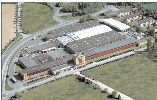
LOROWERK, Bad Gandersheim, Germany
