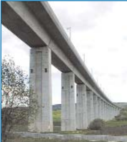
DB Trasse (bridge building)
