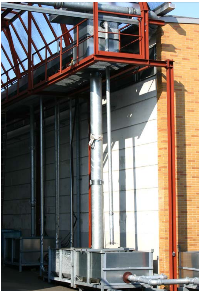
e.g. 100 l drain tower Test field for roof drainage systems with high discharge performance
