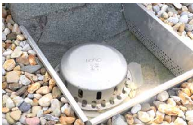
With retention refitted LORO-X RAINSTAR parapet drain
