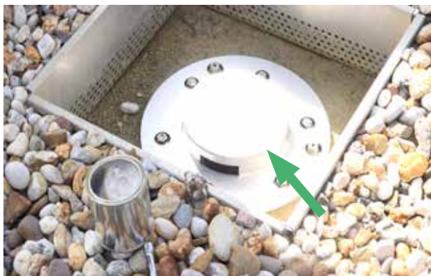
Installation of LORO-X VARIOFIT retention unit
