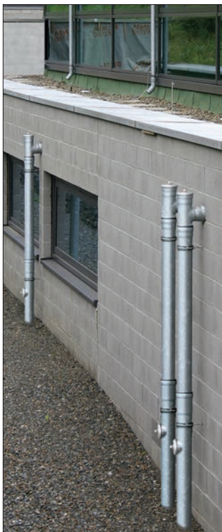
LORO-X rain standpipes and rainwater downpipes with a LORO-X parapet drainage
